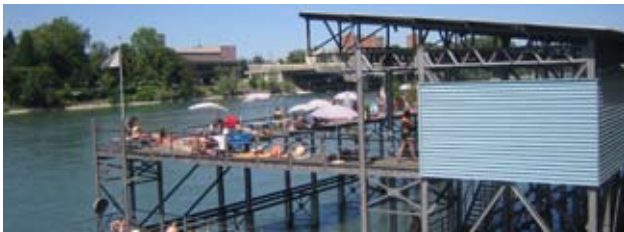
Rheinbadehaus, Basel CH Rhine bathing house, Basle CH
